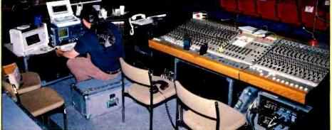
Mixing position at Wembley complete with FFT, EQ rack and computer
