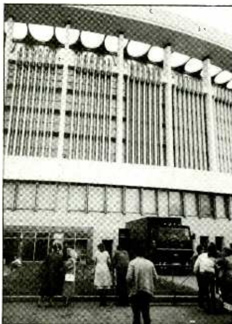
Installed in Leningrad for Billy Joel
