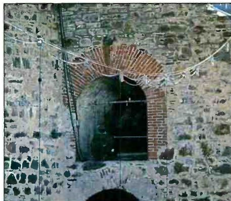
Tamminen's solution: a 50m steel cable between the side walls with a microphone cable support system.
