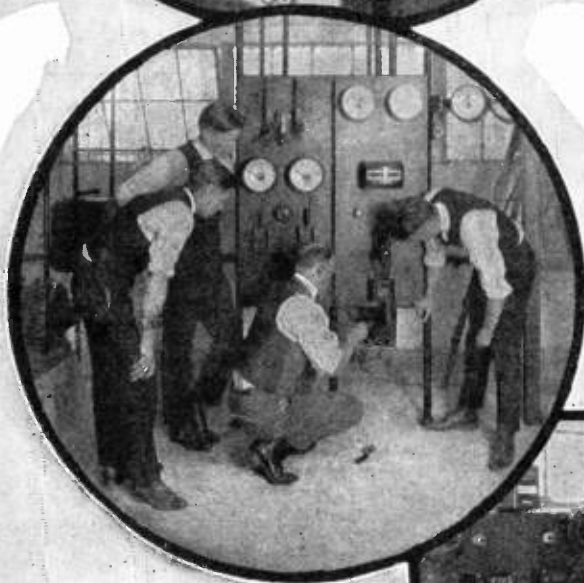
Above. Inspecting construction of switchboard and automatic circuit breaker in C. E. W. Laboratory. Right: View along west wall of C. E. W. Laboratory.
