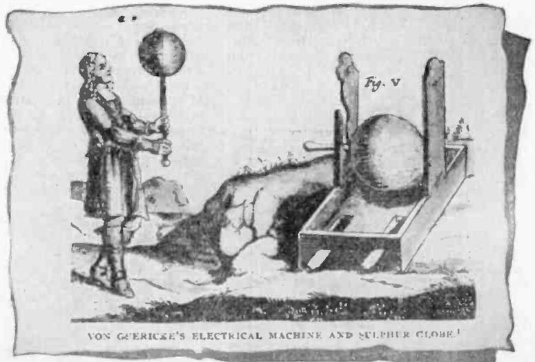
Here the primitive frictional electric machine with no multiplying gear is shown, and the experimenter, carrying an excited ball of sulphur, is driving a feather about through the air.
