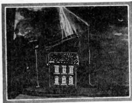
A model of a house is exposed to a Tesla coil discharge to simulate lightning. A little aerial protects it, and no harm is done.
