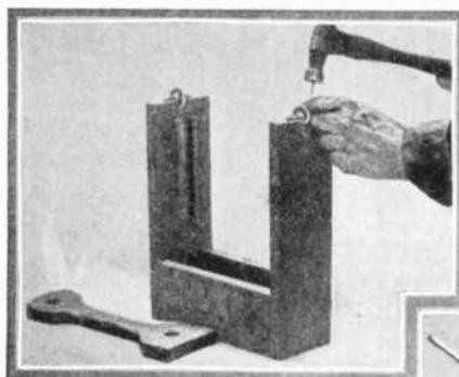
The two cuts on the left show the frame of this battery with pulleys, so as to constitute a plunge battery in which the plates hold their positions in or out of the solution.
