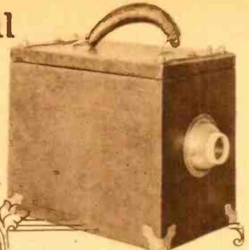
Portable X-ray apparatus, weighing only 20 pounds, developed by Dr. Coolidge and his associates for general use. It is plugged into the regular house circuit.
