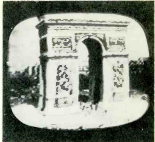
TEN FEET AWAY, PICKED UP ON RABBIT EARS this is the signal the one-third unit produced operating on 18 volts of battery power! Unit will run up to a year without attention or power (other than battery) if properly mounted and protected.
