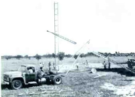
According to Jimmy E. Davidson, manager of the system, Newport Cable is using its own poles. More than 1200 poles are already in place with more than 50 amplifier locations being installed. Nearly one million feet of cable is being used and the system operates from a 420 foot tower with 520 antenna elements.
