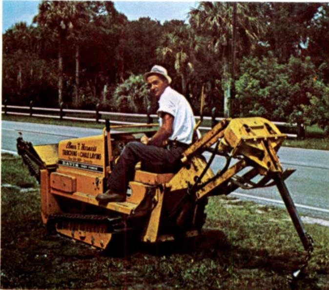
*Use of a vibratory plow for direct burial of trunk and feeder lines is big improvement over trenching.*
