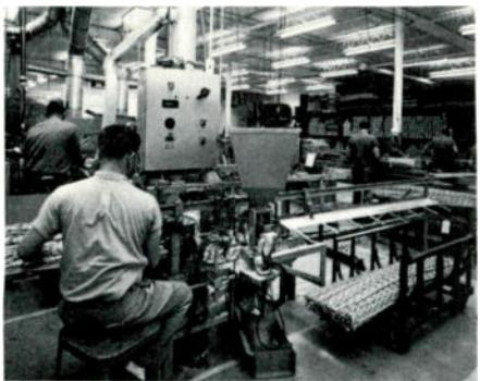
As finished "sets" pass through this machine, inside surfaces of the units are sprayed with a quick-drying adhesive, then coated with a special grit to increase the holding power of the hardware.
