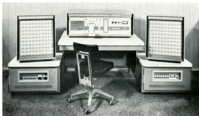
*The production of sophisticated electronic gear for surveillance is on the upswing. The Digitor-400 shown here is a device for monitoring data acquisition and control functions. It can monitor 1,000 sensor circuits over carrier channel.*
