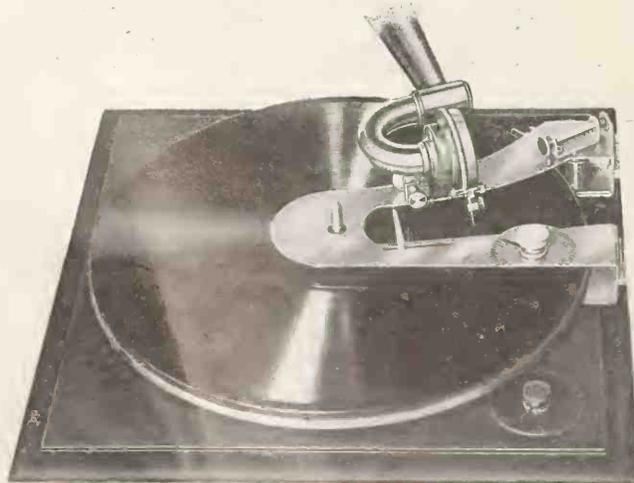
**T**HE SMITH REPEATOSTOP is an efficient "stop" with the added feature of repeating the record once, twice or three times as desired.
