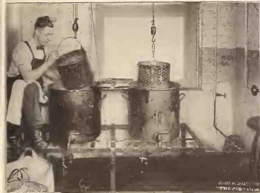
100,000 needles in each dripper are being immersed in chemically prepared bath at 380 degrees of heat.
