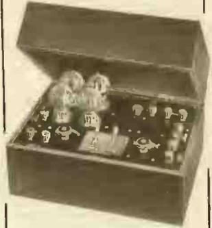
Cut showing typical single tele-megafone set for public speaking—speaker does not have to hold transmitter and is free to walk about.
