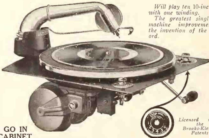
Will play ten 10-inch records with one winding. The greatest single talking machine improvement since the invention of the disc record.
