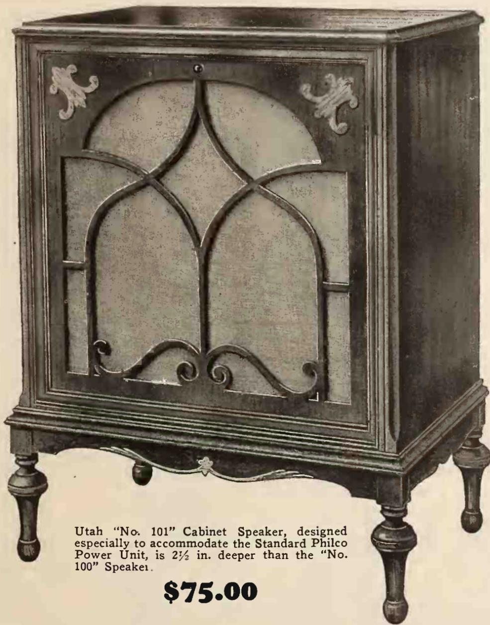
Utah "No. 101" Cabinet Speaker, designed especially to accommodate the Standard Philco Power Unit, is 2½ in. deeper than the "No. 100" Speaker.
