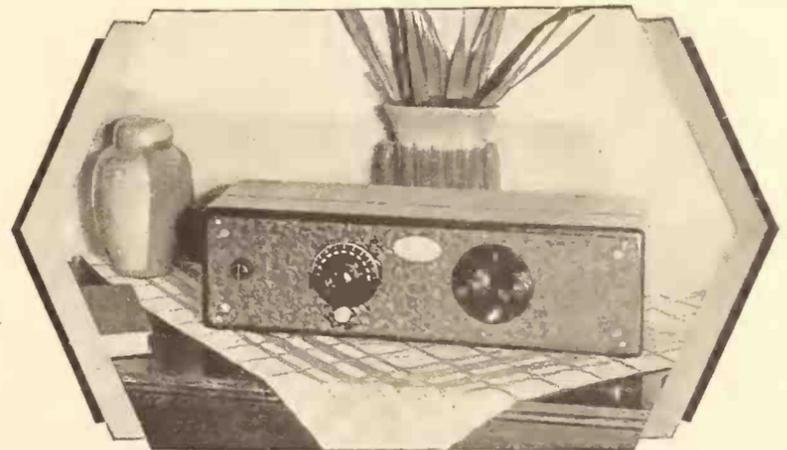
**MODEL 49** battery set. Solid mahogany cabinet. FULL-VISION Dial. Antenna adjustment device assures unusual selectivity. Three stages of T. R. F., detector, two stages of A. F. Six tubes required. **\$68**
