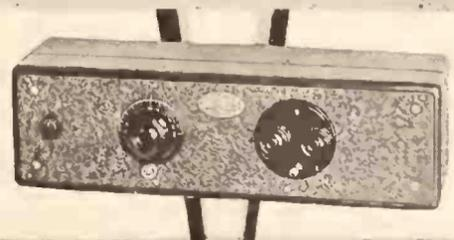
**MODEL 49** battery set. Solid mahogany cabinet. FULL-VISION Dial. Antenna adjustment device assures unusual selectivity. Three stages of T. R. F., detector, two stages of A. F. Six tubes required. Without tubes or batteries, **\$68**
