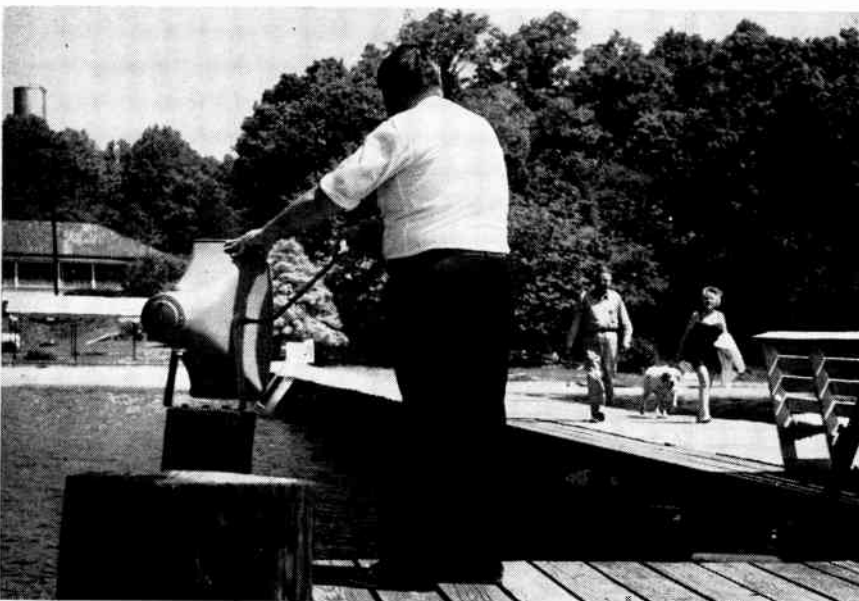
A CDP has been mounted on a pier piling and is being adjusted to cover the beach area about 130 feet away. In the vertical position of the horn, CDP's horizontal pattern is wider (90 degrees for the highs, 120 degrees for the lows) than it would be if mounted on its side. Adjustment of speaker mounting angle is maintained by two nuts, which an ordinary auto lug wrench fits.
