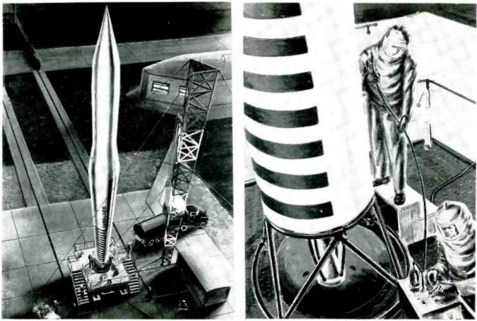
Lett, the Vanguard rocket looks like a giant rifle bullet. Its payload will be a 20 inch sphere crammed with scientific instrumentation. To enter the orbit the satellite will have to obtain a velocity roughly ten times as great as that of a high powered rifle bullet. Right, fueling the rocket is a delicate task. Several of the liquids used in Vanguard are corrosive or inflammable and men must be dressed in protective clothing.
