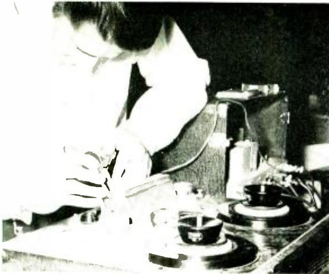
Before the start of each session the recorder heads are cleaned and demagnetized—a practice most tape recordists could follow to advantage.
