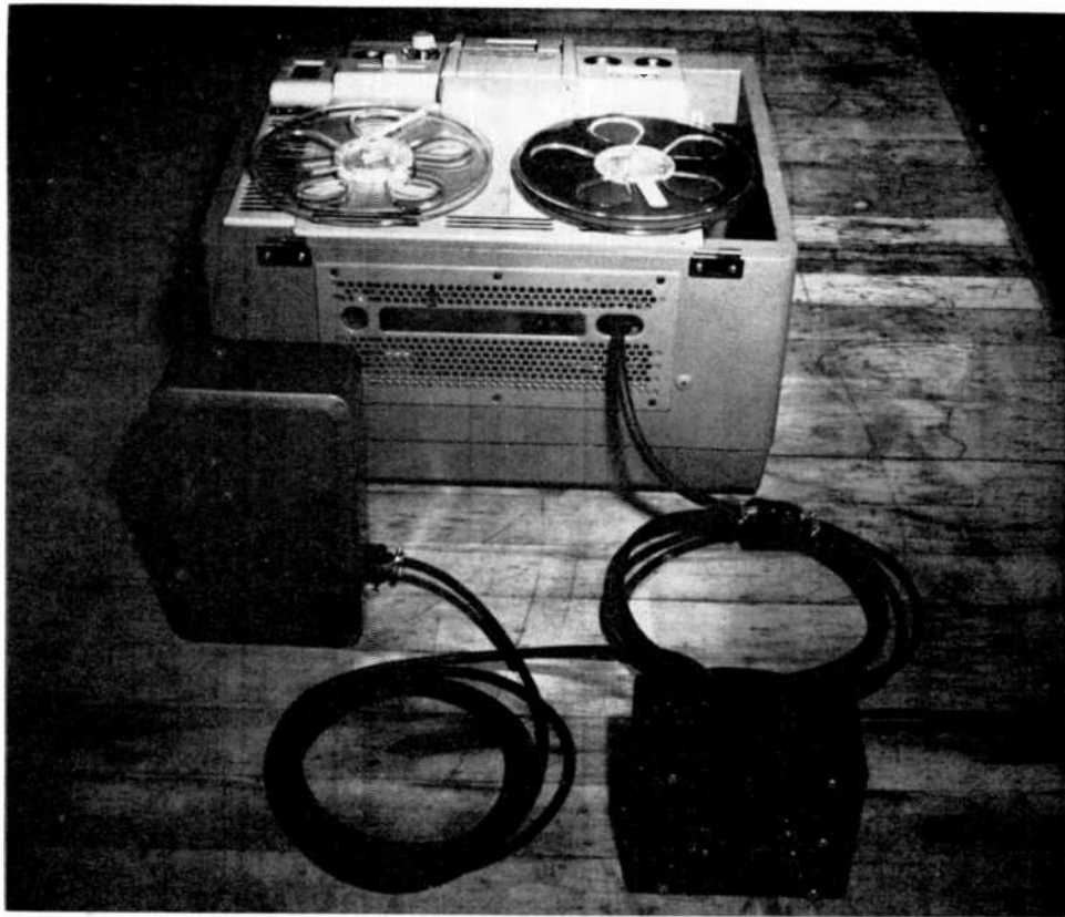
Figure 1: This is the complete system: the control station, lower right, operates the recorder from a remote location. In addition, the automatic timeswitch, lower left, provides automatic cycling.
