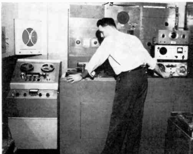
Ed Moravek multiplying the originally recorded pulses. Magnecorder on right is playing back a double speed, Ampex at left is recording at slow speed. Process is then reversed to double the frequency again.
