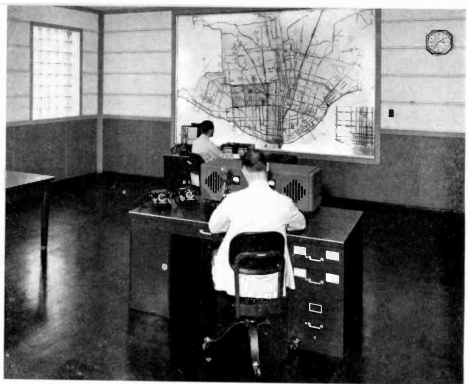
The main transmitter (left) for the St. Louis Public Service Co. Radio Station. This unit, which is unattended, is remotely controlled by the console in the dispatcher's quarters (shown above). The illuminated map shows the entire street car and bus system of the company. It is divided into ten districts by means of different colors, each district being under the supervision of one of the radio cars.
