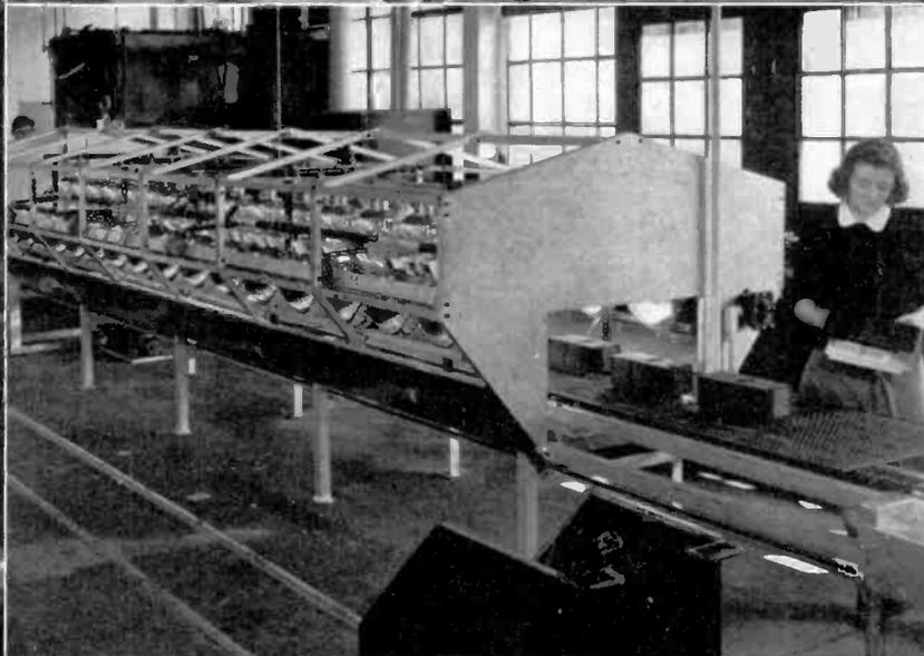
Infra-red baking tunnel at Western Electric's Kearny plant cuts 75% from drying time on wrinkle-enamelled aircraft radio housings. Sixty-four lamps consuming 60,000 watts heat steel of housings to 425°F. At left, new type jig for slitting quartz crystals eliminates scratches, speeds production, and reduces breakage about 75%. Jig is shown in use by its designer, Benjamin Willett, instructor in crystal laboratory of RCA's Camden plant. Four or five 8-meg blanks can be cut at one time.
