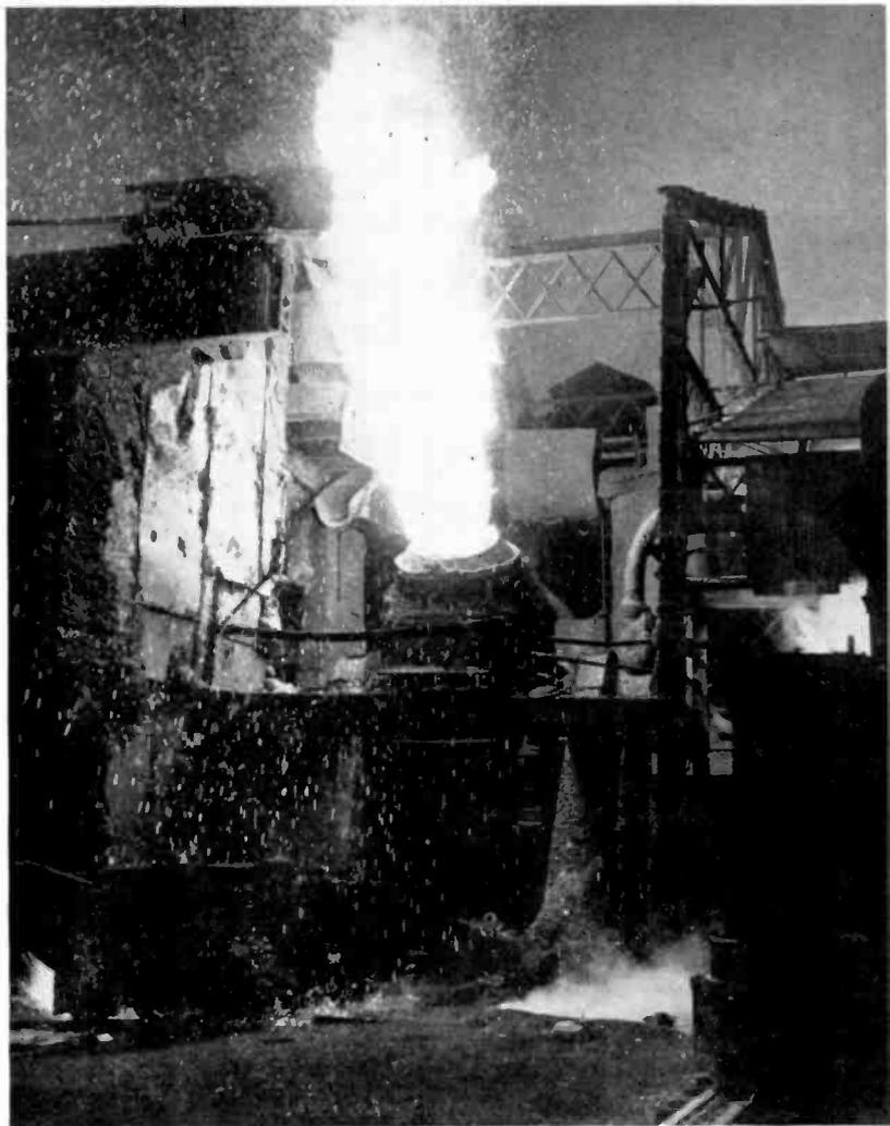
**Bessemer early in steel cycle, before photoelectric control has operated. See front cover for later stage**
