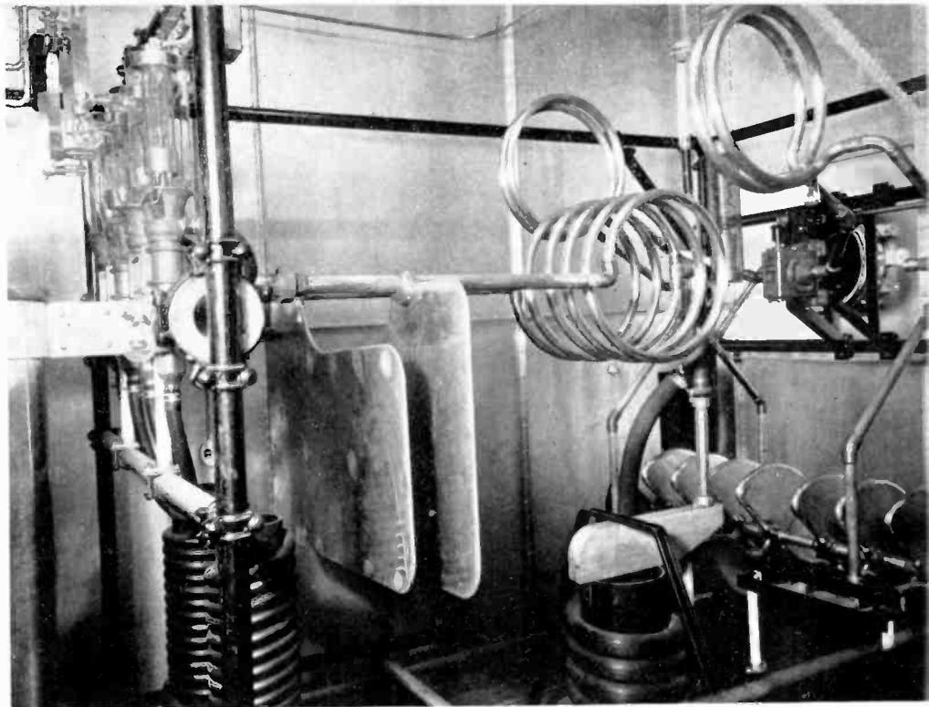
Power stage of "Thermex" 60 kilowatt high-frequency electrostatic heating equipment. Note tubes, tank circuit, and coupling coils
