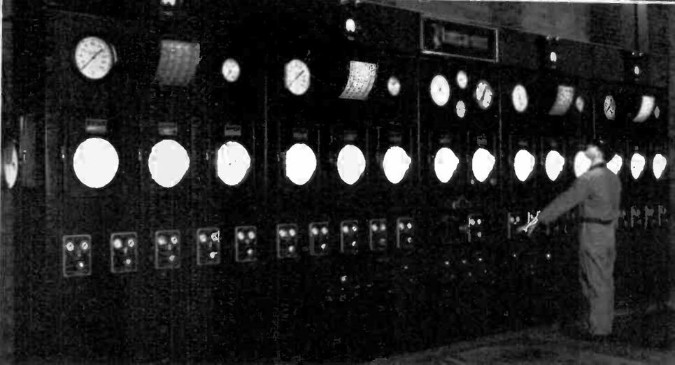
At right, sensitive photo-cells indicate combustion efficiency by measuring density of haze in smoke stacks to one-half of one per cent CO<sub>2</sub> variation. Picture is boiler room of Parkchester Housing Project, Bronx, N. Y., showing four Ess Haregases (top of pane) and eight-pen recorder (at extreme left).
