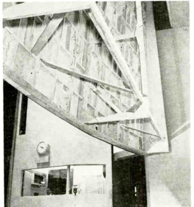
**CONSTRUCTION DETAILS** are seen above of the heavy drop. Below, the elevation sketch of the stage shows how the exponential-horn form has also been applied to the vertical section of the new WOR theater studio
