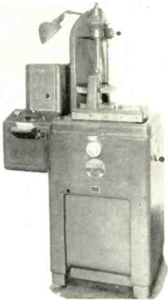
INVOLUTE MEASURING machine equipped with GE chart type electronic recording device manufactured by Fellows Gear Shaper Co.
