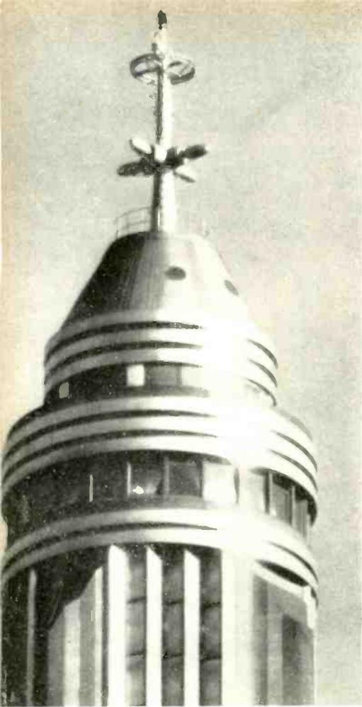
WNBT - W2XWG ANTENNAS. Lower turnstile elements simultaneously transmit television pictures and FM broadcasting without mutual interference
