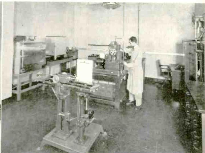
**INDIVIDUAL LABORATORIES** are completely equipped for the investigation of particular projects. In the one above, an investigation of the physical properties of rubber is under way. Tensile, compression and plasticity tests are conducted here on rubber compounds under controlled temperature and humidity conditions
