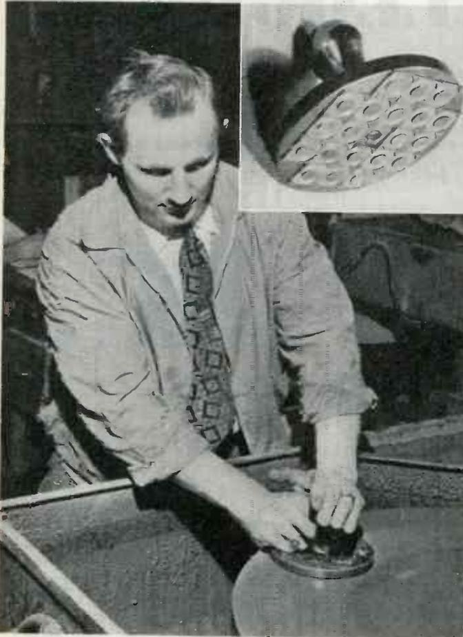
**LAPPING FIXTURE** holds twelve electrodes. By adopting technic used to lap crystals themselves, RCA Camden plant cuts electrode lapping time to 0.8 minutes from old hand-lapping time of 2.0 minutes each. Close-up at top right
