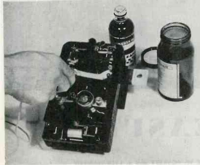
**LOCAL SILVER-PLATING** of electrical equipment to reduce contact resistance with portable apparatus developed by Rapid Electroplating Process, Inc., 1414 So. Wabash, Chicago. Powered by rectifier or battery, swab-like applicator anodes are used, with electrolytes for silver, gold, zinc, copper, nickel, tin, or cadmium plating
