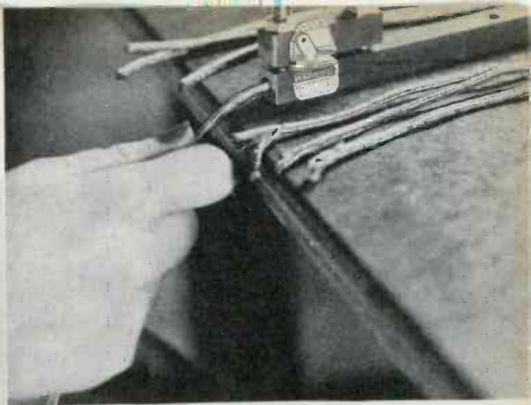
**SHIELDING STRIPPER** cuts time of operation from 55 seconds to 15 seconds at Submarine Signal Co., Boston, Mass. Wire is inserted, then pulled out. Pawl-action knife cuts metal braid. Screws adjust for length and depth of cut
