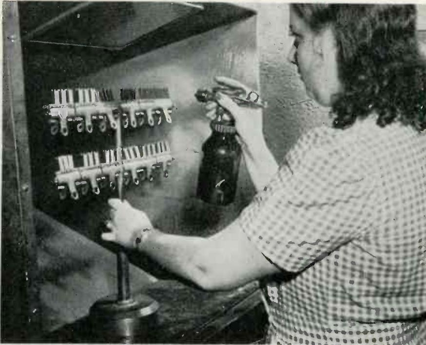
Graphiting tube anodes by spraying with suspension of graphite in water, at RCA tube plant
