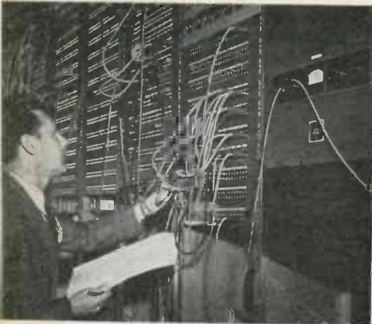
Part of patching equipment which occupies one side of master control room
