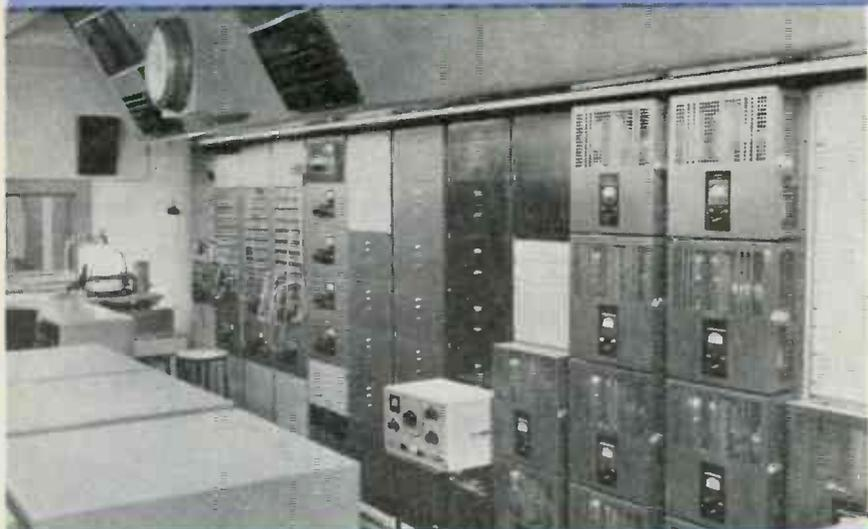
Opposite side of the recording room, containing thirteen racks of equipment, holds 46 Western Electric amplifiers of various types. Partial view of the master control console in the recording and transcription room. Turntables work in pairs with automatic switching.
