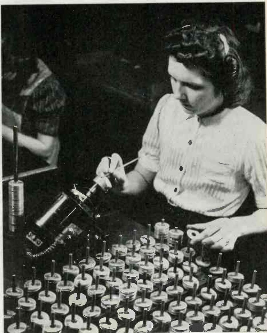
Coating disks for copper-oxide rectifier cells with colloidal graphite improves efficiency by insuring intimate electrical contact, at Westinghouse, East Pittsburgh, Pa.
