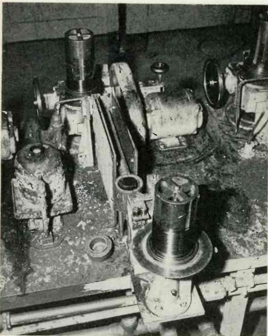
Tungsten wire for vacuum tube filaments is drawn to size through diamond dies lubricated with colloidal graphite in RCA Harrison, N. J. plant
