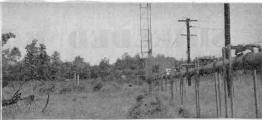
Power is fed to the tower through a feeder system extending several hundred feet to the transmitter house. The gin pole, hoisted together with its fastenings to the top of the tower, is in two sections, assembled on the ground.
