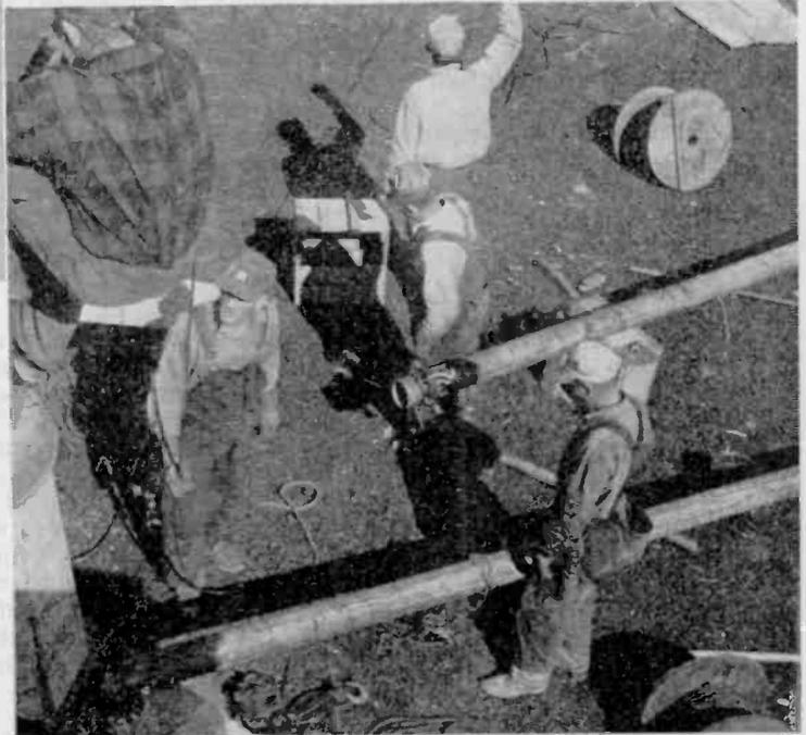
Approximately 150 tons pressure is supported by the base insulator, representing weight of tower and strain on guys; this bottom section is not dismantled but is merely unbolted from the foundation and transported to the new location.
