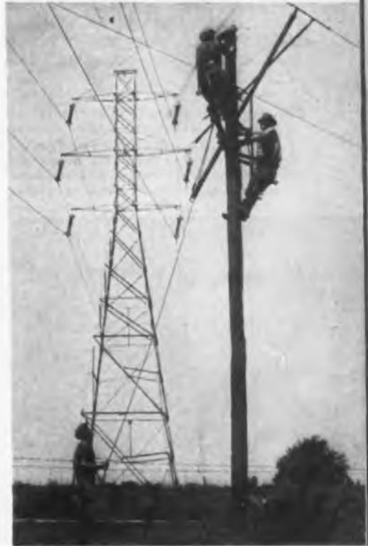
Fig. 6—Linemen, replacing insulator on 6.9 kv line, can be called in emergency by space radio
