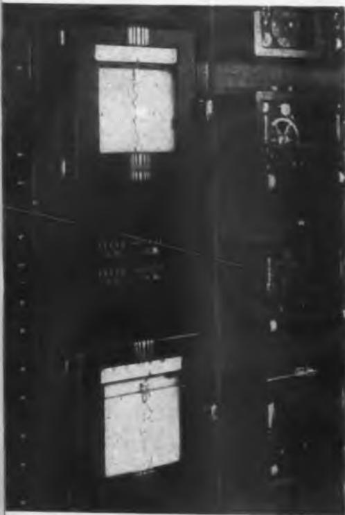
Fig. 9—Main switchboard at Winfield hydro plant. First four panels contain supervisory control equipment for operating this plant from Turner station. Carrier equipment installed outdoors at both locations
