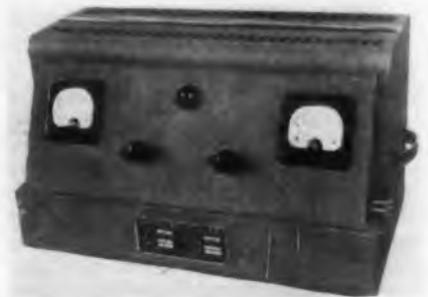
Typical laboratory rectifier unit for plug-in operation from 115-volt single phase supply
