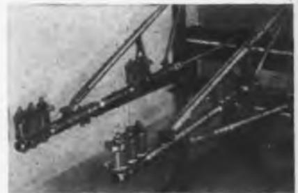
AIRCRAFT IN-LINE ENGINE MOUNTING
