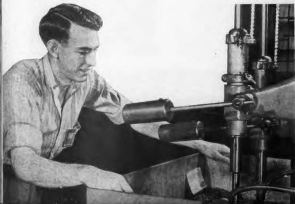
**1V** STRIPPING enameled wires for soldering. New method at Electronic Laboratories, Indianapolis, Ind., is twice as fast as old way and lengthens life of wire brushes in motor-driven stripper. Solder pot at right, filled with molten lead, softens enamel before brushing.
