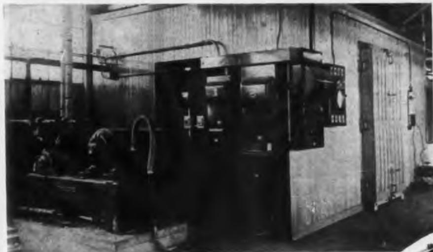
**8** ↑ **TEMPERATURE CHAMBER** one of the largest ever built, accommodates all units of a complete radio range station for test at the Aerial Navigation Division of Federal Telephone and Radio Corp., Newark, N. J. Inside measurements are 22 1/2 by 19 ft. high. Range is 55 degrees C. down to minus 30 degrees C. in little over 20 minutes
