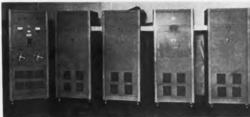
Group of selenium rectifier units, with master control panel at left end, to provide output of 1500 amperes at up to 48 volts
