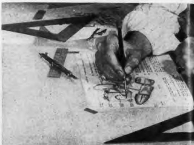
1. Above: Short cuts to worker training are graphic charts used in Westinghouse electronics laboratories and experimental factory for tube production. The picturizations represent a technic borrowed from correspondence schools. Some jobs are done at sight by the use of the charts, all are standardized
