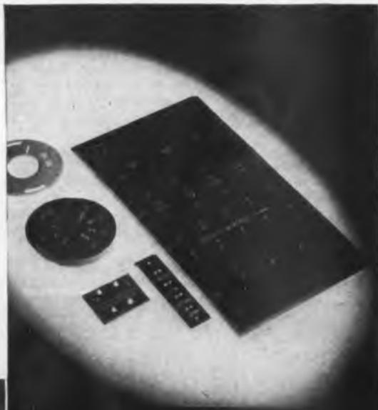
In instruments of communications of every description, parts of National Vulcanized Fibre and Phenolite, laminated Bakelite, have extensive and varied use. These possess great dielectric strength, lightness in weight and exceptional wearing qualities.
