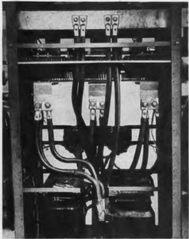
On this large rectifier unit all connections are of the permanent indent type. View shows only terminals; but Indent connectors are also available for end-to-end as well as detachable connections.
