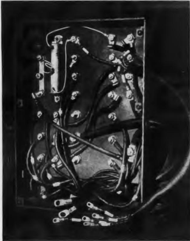
All connections in this panel on Diesel generating unit are made with Burndy Indent connectors, both the straight barrel and the right angle types being used.
