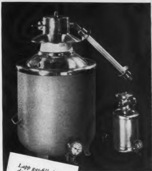
Lapp gas-filled condensers provide zero loss, high capacitance for small space requirement, non-failing puncture-proof design, constant capacitance under temperature variation.
