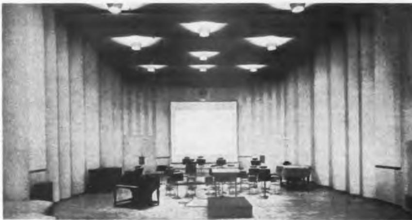
Front view of the scoring stage showing the use of curved plays of different diameters around walls, designed to control reverberation and sound decay
