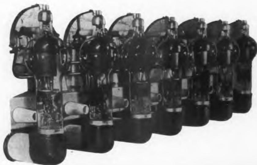
**CLOSE-UP** of the 12-kv rectifier installed at Station WABC, Columbia Island, and manufactured by Federal Telephone & Radio Corp., an affiliate of IT&T
