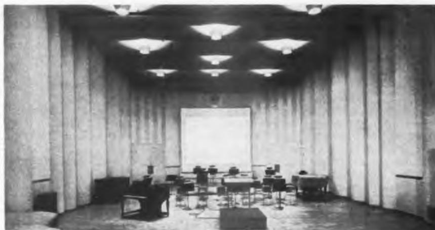
Front view of the scoring stage showing the use of curved splays of different diameters around walls, designed to control reverberation and sound decay
