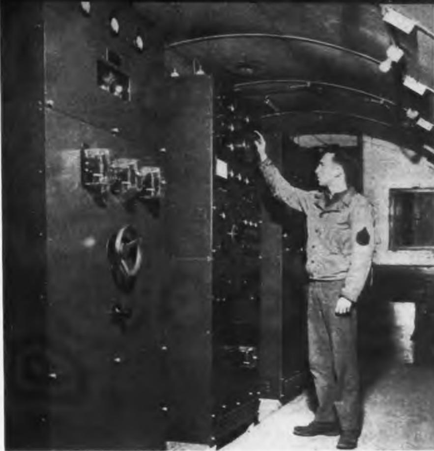
Installed in a Nissen hut in Iceland, this combination of an R-339 and BC-340 transmitter is capable of a total output of 10 kilowatts
