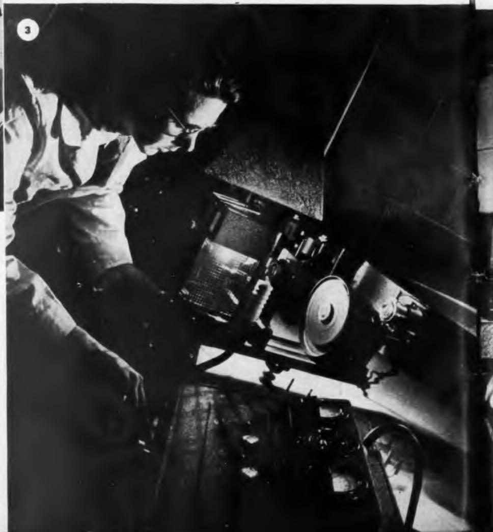
1. Development tests being run on a new type of welding timer unit involve the use of a large mercury vapor rectifier tube
