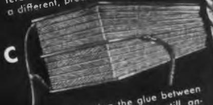
This job of heating the glue between layers of plywood requires still another totally different combination of power and frequency. Unlike A and B this is not induction but dielectric heating—in which the heat is generated within non-metallic substances.
