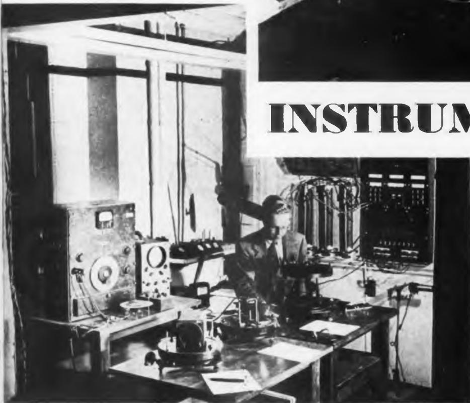
3. Attitude gyro, a new instrument designed to give exact visual indication to the pilot of the plane's attitude—whether it is climbing, diving, or banking. Operator shown with stroboscope checking behavior of an attitude gyro rotor on bench. Complete unit shown on right
