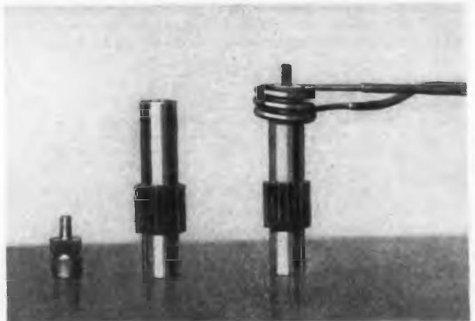
**TO HARDEN CAM SURFACE BY INDUCTION HEATING.** (Below right). Time: One second. Results: Cams were file tested and found a good wearing surface to a depth of .015 in.
