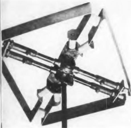
Fig. 3—One of localizer beam radiators for producing pattern shown in Figs. 2 and 4
