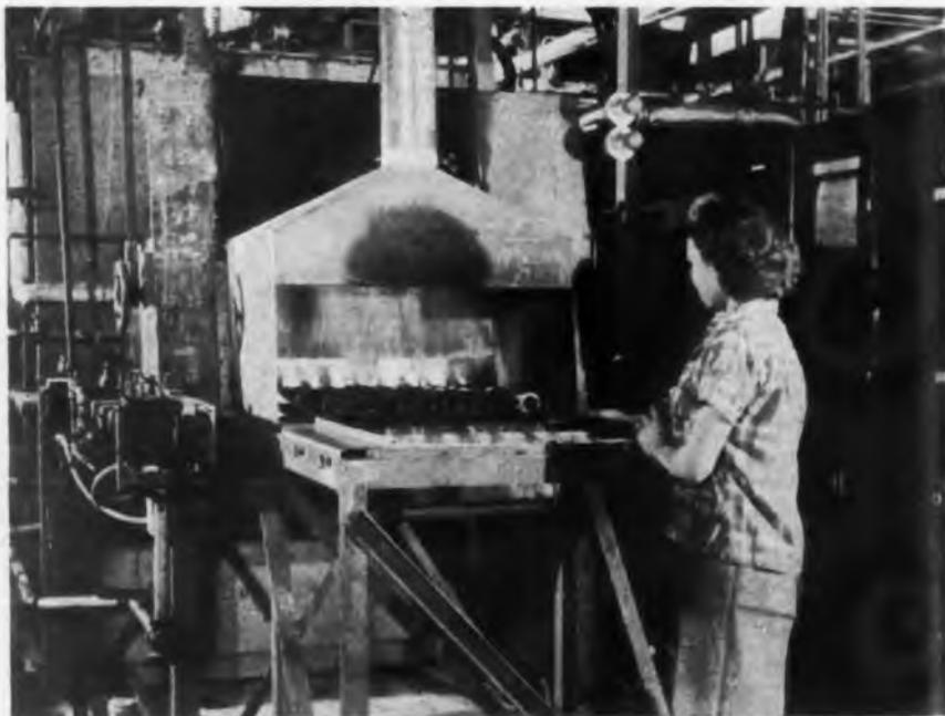
A new job for photoelectric door openers enables unskilled labor to do a good job in the plant of Burgess-Norton Mfg. Co., Geneva, Ill. The installation was made on a new-type, triple action, automatically controlled furnace which brazes, heat-treats, and quenches tank-track parts. The photo is a close-up of the furnace feed. A timer sets the feed-rollers in motion, carrying a tray of parts toward furnace door. The tray in-
