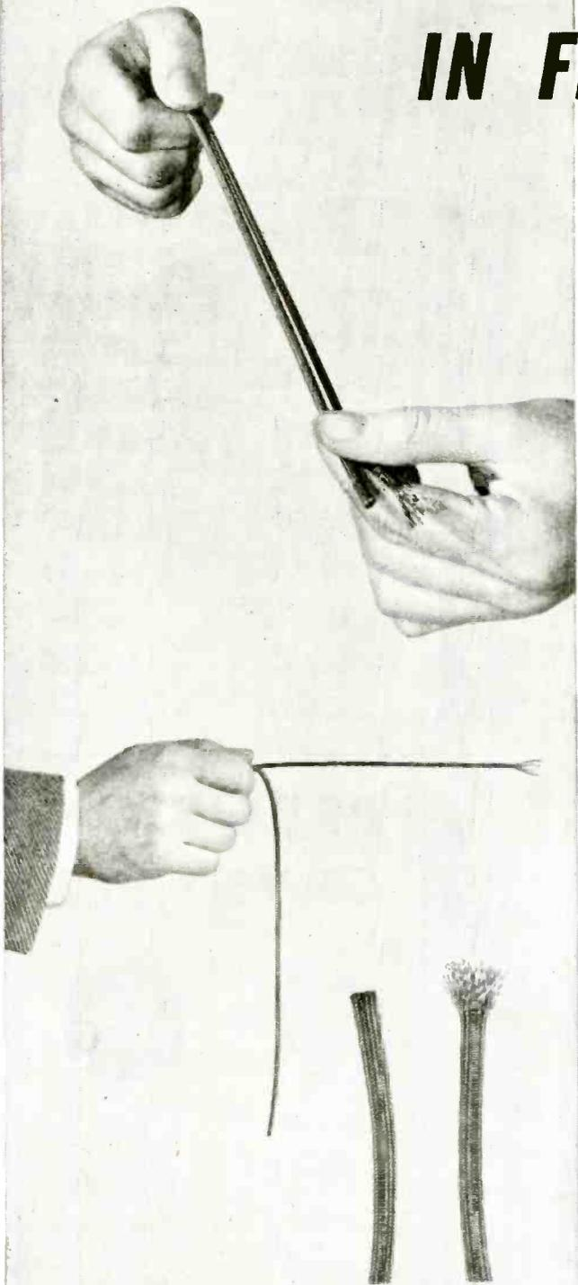
**That new BH Fiberglas "extra Flex" Sleeving is more flexible than saturated sleeving**
