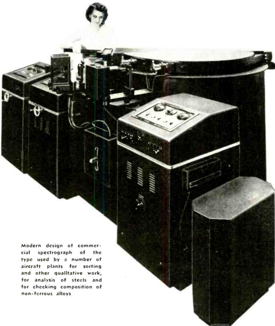
Modern design of commercial spectrograph of the type used by a number of aircraft plants for sorting and other qualitative work, for analysis of steels and for checking composition of non-ferrous alloys
