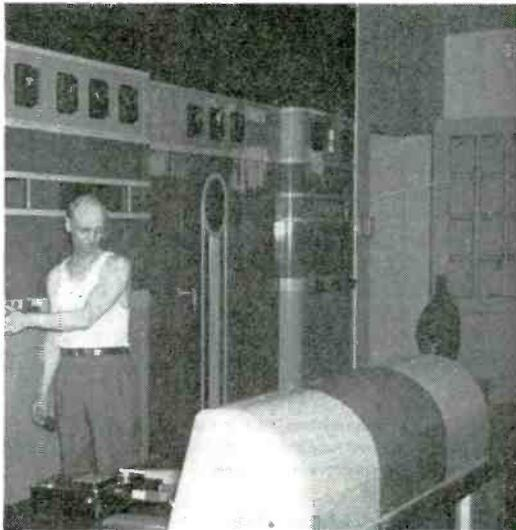
WJZ. The three NBC-built transmitters are in the enclosure with audio and controls between them
