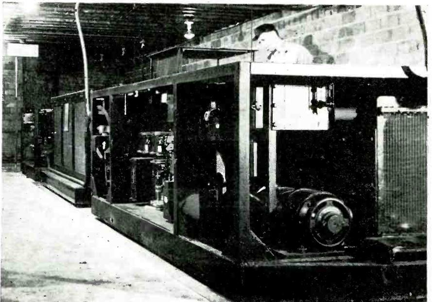
Dc end of Ignitron unit in coal mine showing water-to-air heat exchanger for cooling tubes
