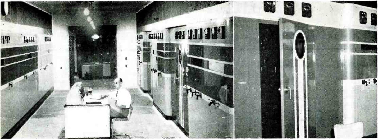
The three RCA transmitters, shown above together with the console that controls them, are located in the wing of the building formerly occupied by wing at the back. Right, above, one of the technicians adjusts No. 4 for operation. Transmitters have duplicate radio frequency channels, at ends of
