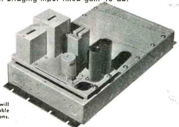
The 3A Mounting Frame, requiring 10½ inches rack space, will accommodate up to THREE 102 Series Amplifiers and is suitable for wall mounting cabinet or rack and panel installations.
