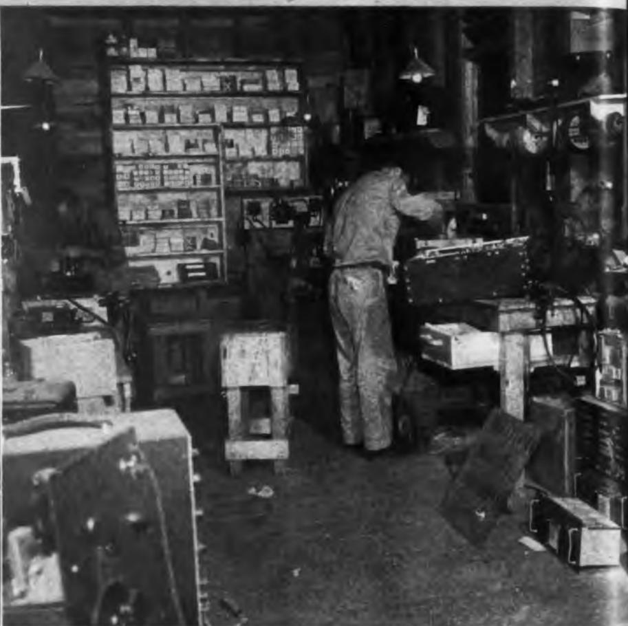
Left—The "first echelon". Radio operator himself can tune up, replace tubes, and make "screwdriver adjustments" in his radio gear. Right—A third echelon stationary radio repair base, showing somewhat larger stocks of replacement tubes and parts available. Here servicing is an exact science
