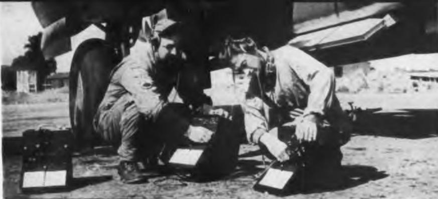
Daily preflight check on transmitter and receiver field strength, sensitivity, and frequency
