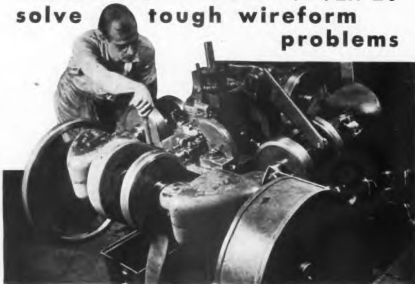
**D**ID you ever see a fourslide in operation—turning straight wire into intricately-shaped wireforms with each combination stroke of its four slides? If you have, then you know the skill and experience that is necessary to set-up these machines—to put them in operation for high production of unusual round and flat wire shapes.
