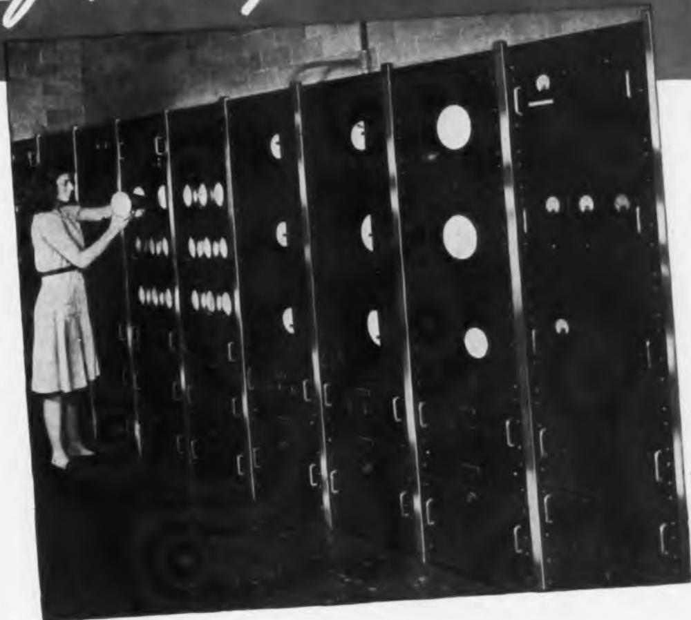
One of the most elaborate cathode-ray tube test racks in this country operates day and night, seven days a week at National Union. For, at N. U., cathode ray tube production
