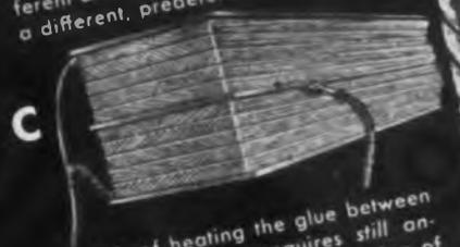
This job of heating the glue between layers of plywood requires still another totally different combination of power and frequency. Unlike A and B this is not induction but dielectric heating—in which the heat is generated within non-metallic substances.
