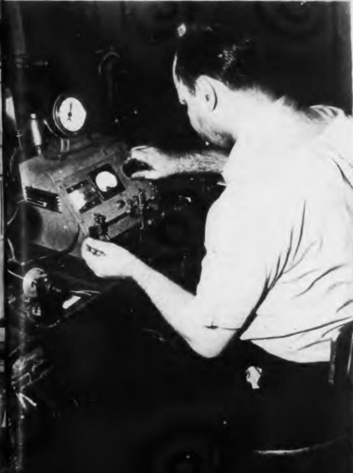
**7 PINHOLE DETECTOR** for enameled wire was developed at North American Phillips Co., Dobbs Ferry, N. Y. Wire runs through two mercury pools held at 500 volts dc. Any conduction actuates electronic relay and counter. Checks lengths 1/4 to 8-in., or continuously
