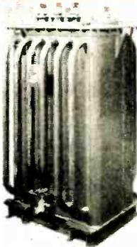
150 KVA Distribution transformer, single phase, 600 high voltage, 240/120 low voltage.
