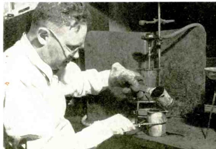
Firing of experimental ceramic samples in determining the relationship between composition of material and its characteristics
