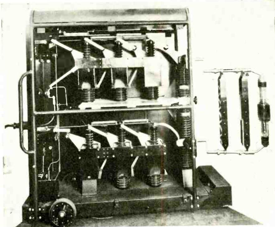
Fig. 3—Marx circuit surge generator for Westinghouse high speed X-ray tube
