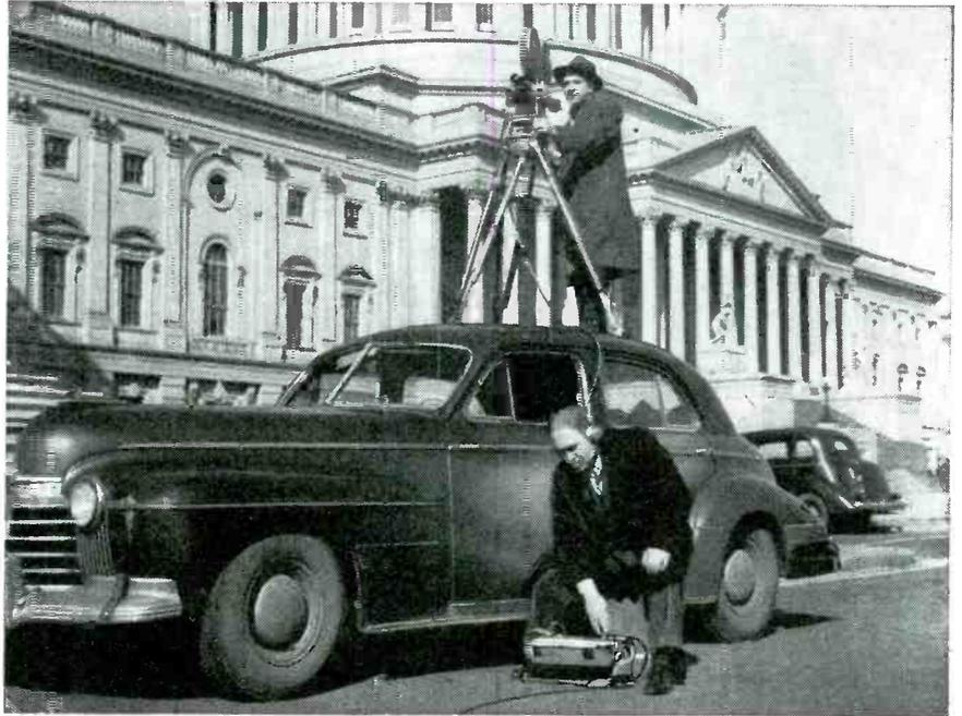
PORTABLE SOUND EQUIPMENT used by Pathe News' Washington staff must be ready for instant action, rain or shine. To meet all requirements of newsreel work, Pathe News engineers developed a lightweight sound amplifier—powered by a special, flat type 180-volt Burgess Battery—with sufficient output in milli-watts to operate the mirror galvanometer. Burgess engineers worked closely with Pathe sound experts to develop this battery (photo lower right).
