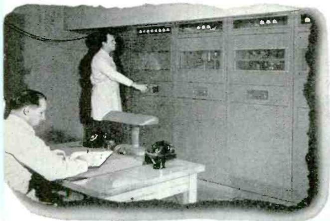
Grid modulation is employed at WBKB and a broad band of frequencies must be passed in all stages following the modulated amplifier. Multiple-tuned resistance loaded coupling circuits are used between stages.
