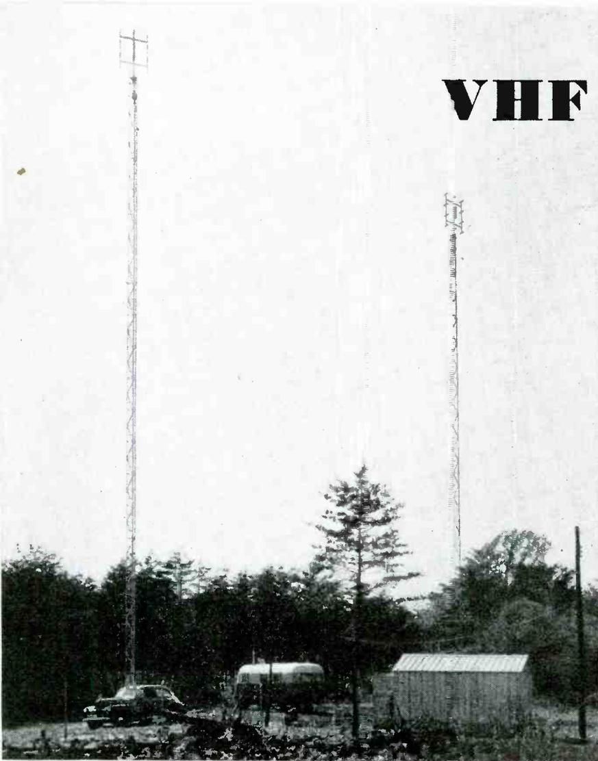
Fig. 2. The 24-dipole receiving (left) and transmitting (right) arrays used at Arlington, Vt., relay site
