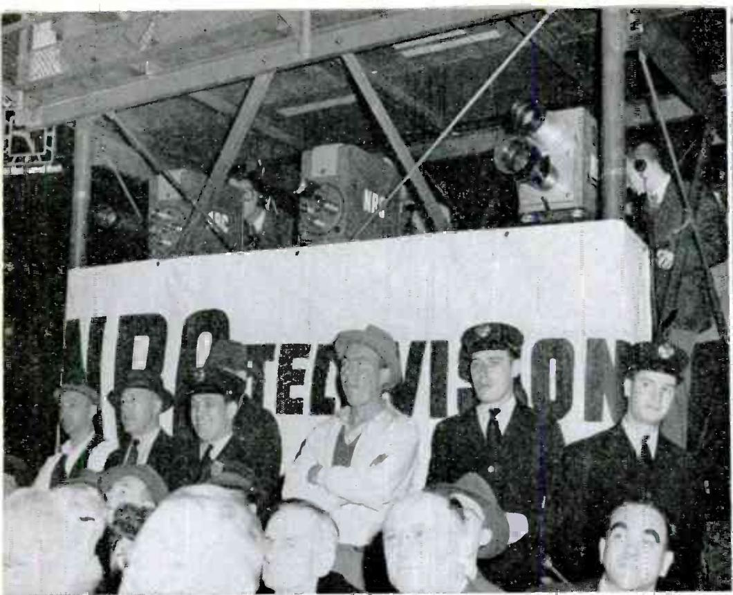
Close-up of the NBC booth, showing two of the new Image Orthicon cameras in position, alongside an experimental camera used together with two more pre-war Orthicons, five altogether
