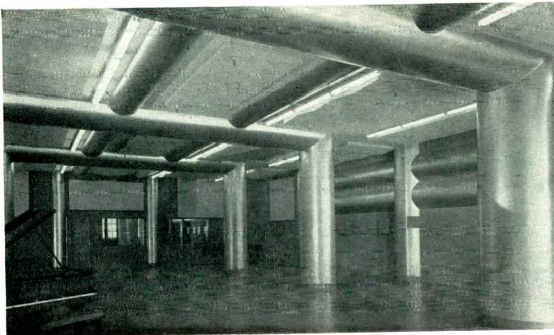
Reeves Laboratory band studio in New York City where some of the sound measurement tests were made. Note the acoustical construction of the walls. Equipment used in recording the tests is shown on following pages
