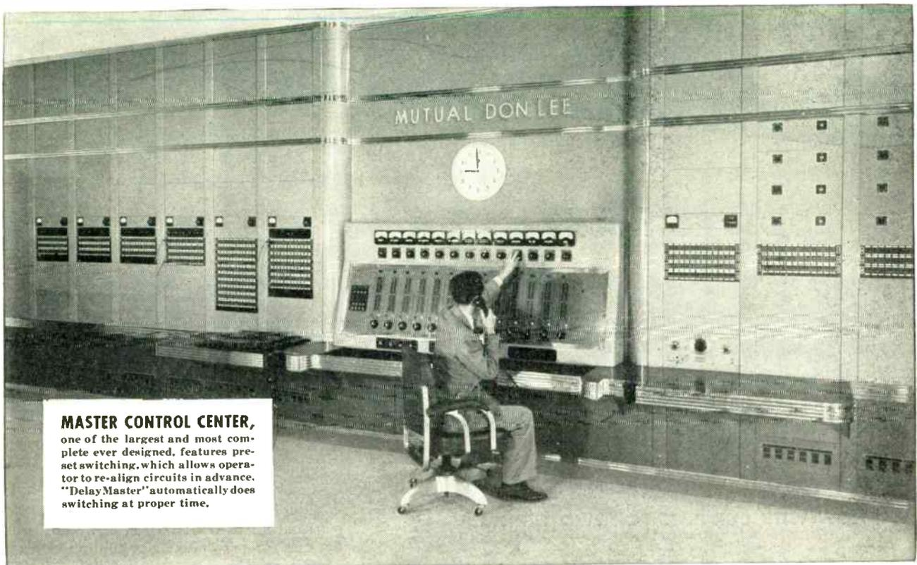
**MASTER CONTROL CENTER,** one of the largest and most complete ever designed, features pre-set switching, which allows operator to re-align circuits in advance. "Delay Master" automatically does switching at proper time.
