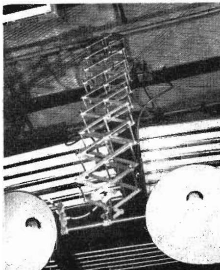
Fig. 10: (Left) Spaced ceiling pantograph units of the type shown provide a flexible method for handling problems of fill light. Fig. 11: (Below) View of lighting facilities installed in NBC's Studio "C", New York
