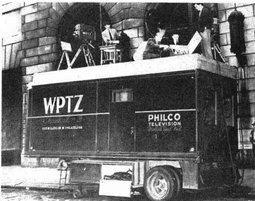
WPTZ, Philadelphia, recently placed in service what is believed to be the first truck-trailer used for mobile telecasting. The tractor-trailer combination eliminates the possibility of serious delays in reaching the scene of the telecast. Should the tractor fail for any reason, another tractor can be immediately coupled to the trailer. The manufacturer (Trailmobile Co., Cincinnati 9, Ohio) claims more space is provided in the trailer than in mobile truck units
