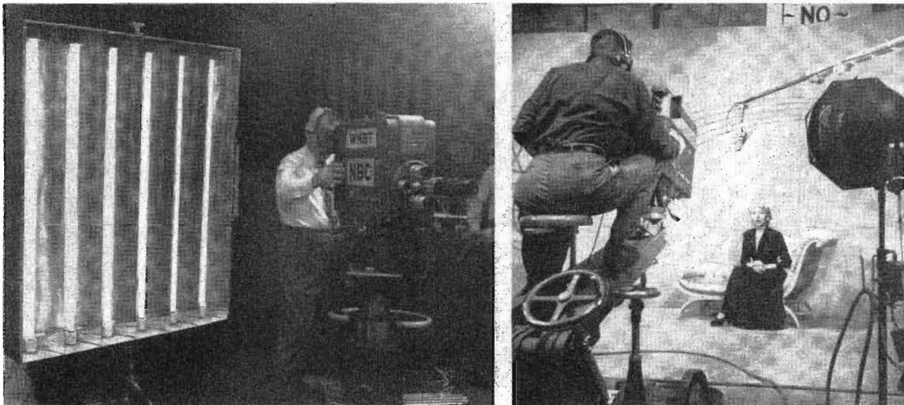
Fig. 12: Fluorescent and filament sources, mounted in stands with large roller casters, are used to complement lighting from ceiling fixtures
