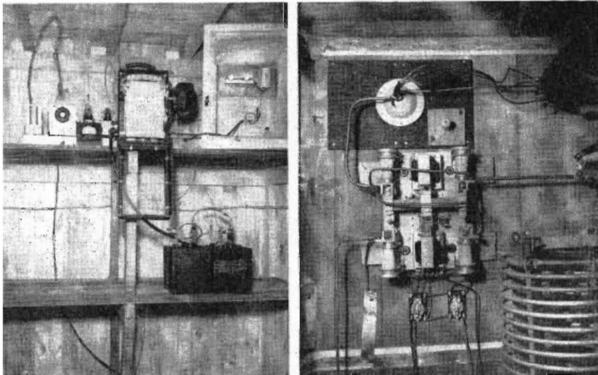
Fig. 3: (Left) View of first working installation shows (l to r) receiving unit vibrator pack, receiver, amplifier control chassis, recording receiver and heated cabinet
