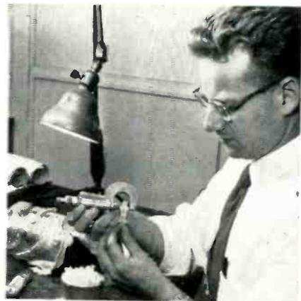
← Possibly the only epoxy casting in the Phila. Metropolitan area, a ph flow assembly component is being poured. It will then be baked in the large Dispatch Oven, Model Y-29-2 (\$650), in rear.
