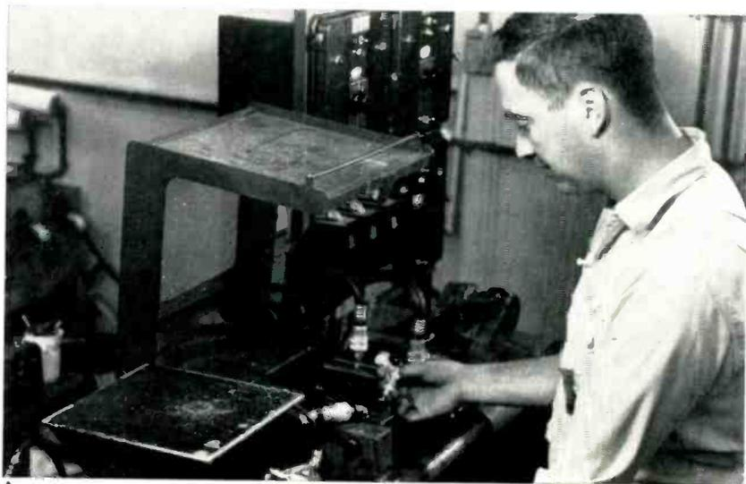
↑ A nylon camshaft, used in L&N recorders, has just been completed in a Van Dorn Injection Molder, 2 oz. Model (\$4,800).
