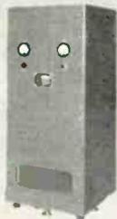
This transistorized MAGAMP power supply delivers a 27V to 42V output at 0 to 300 amperes, regulated at a load up to several hundred feet away.
