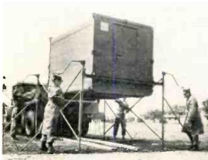
An easily assembled lifting device simplifies the Army's task of raising this Craig Helicop-Hut to level of truck bed. Shelters are designed to house complete radar, microwave or other installations
