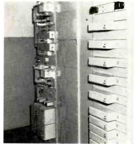
VHF equipment in the toll booth communicates with a base station at the nearest maintenance station, and thence by microwave into the central control console. A short audio tone precedes each transmission originating from a toll plaza, causing a tone receiver in the control console to light an identifying lamp.
