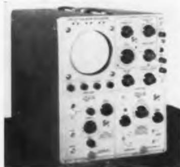
handling versatility. Risettime of the two main vertical amplifiers is 0.012  $\mu$ sec, and both have 0.2  $\mu$ sec signal-delay networks. The Type 551 sweep is common to both beams. It has 22 calibrated direct-reading sweep rates. Amplitude calibrator has 18 fixed steps. Tektronix, Inc., P. O. Box 831, Portland 7, Ore.
