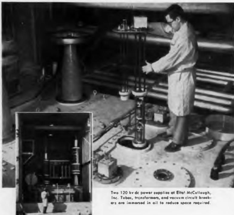
Two 120 kv dc power supplies of Eitel McCullough, Inc. Tubes, transformers, and vacuum circuit breakers are immersed in oil to reduce space required.
