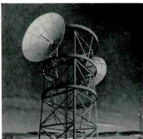
Ring mounts simplify orientation, make future antenna installation easier and less costly.
