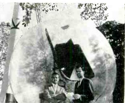
Hughes' E. W. Tempkin and Dr. N. A. Begovich stand in front of novel antenna of their new "Frescanar" radar which simultaneously computes distance, bearing, height.
