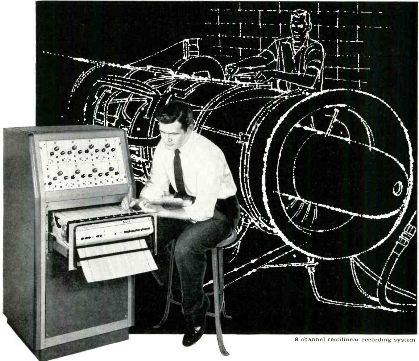
8 channel rectilinear recording system
