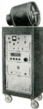
**TV PROJECTION SYSTEM PB-611A** throws bright pictures that can be viewed with equal ease by 100, or more than 1000 people. This versatile TV projector is compact, mobile and completely self-contained. Handles broadcast or closed circuit programming. It projects up to 12' by 16' pictures.
