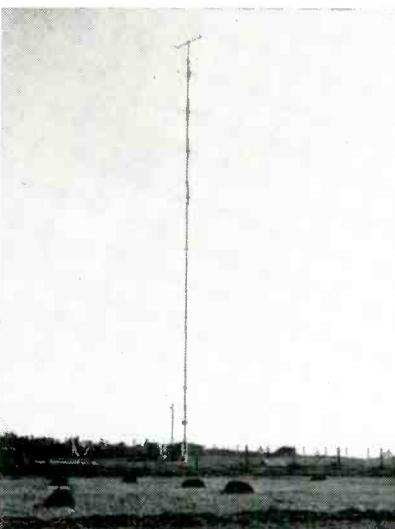
The BBC is using "translator" stations to relay television programs to outlying towns in England. Pictured below is the receiving and transmitting aerial mast on Creteway Down. The television translator units can be seen near the base of the mast.
