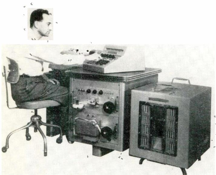
Fig. 2: This tube type computer consumes 18 kw and requires a heat sink. Its transistorized version is shown in
