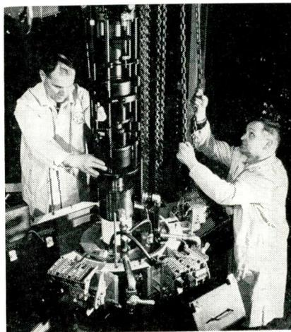
GE technicians install multi-million watt klystron in the FPS-7 super power radar
