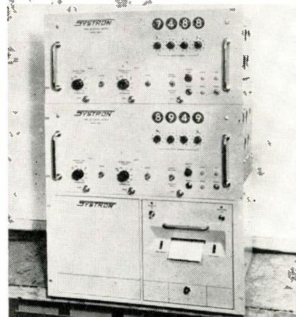
Model 1021-1 time interval meters take simultaneous measurements of elapsed time between the emitted signal and the return signal from two different ground stations. A Systron Model 1401-1 digital recorder provides a permanent printed record of both times and identifying code. Features include Nixie in-line readout, direct readout in nautical miles, and automatic subtraction of fixed delays. Systron Corp., 950 Galindo St., Concord, Calif.
