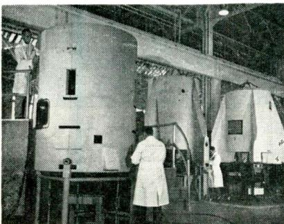
Tail sections for the ballistic rocket that will carry man into space are nearing completion at Reynolds Metals, Sheffield, Ala.
