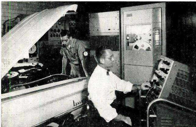
Knock, pre-ignition, rumble, and thud are ferreted out by this equipment, developed by Du Pont Co. and installed in their Petroleum Laboratory.
