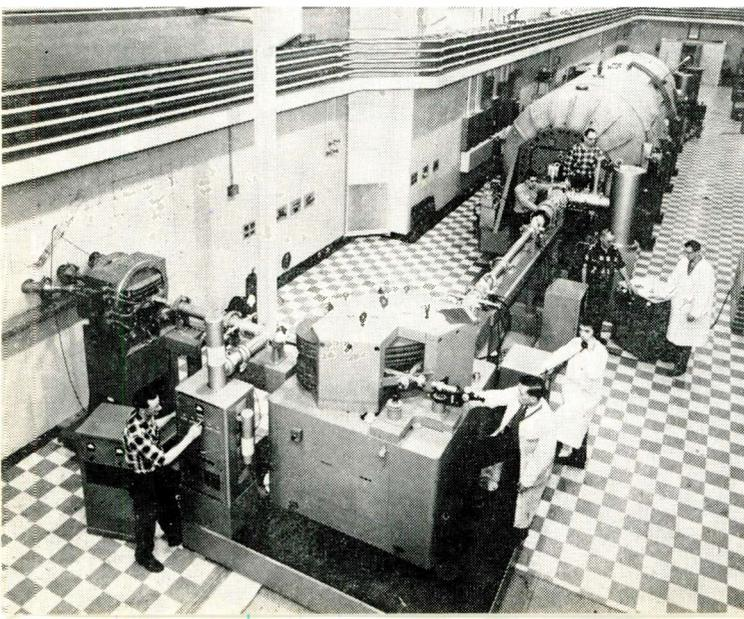
Tandem Van de Graaff particle accelerator, a 10-million-electron volt research tool built by High Voltage Engineering Corp., Mass., will be used in basic nuclear research by the Danes.
