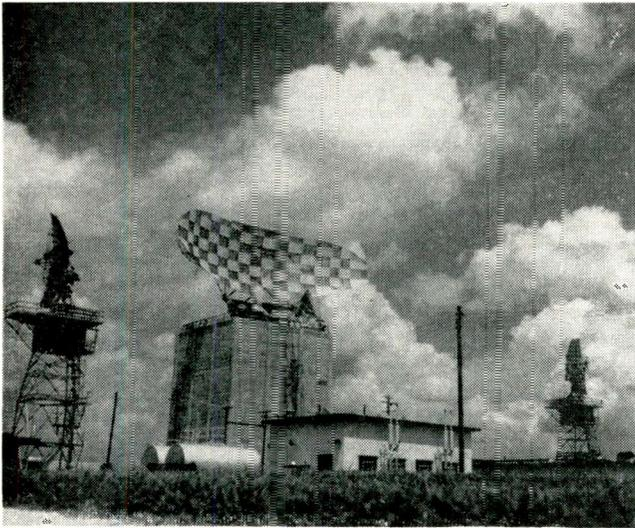
The Air Force's AN/FPS-35 shown at Thomasville Aircraft Control & Warning Site, Alabama. Sperry Gyroscope was system manager. Antenna weighs nearly 70 tons. Tower is 85 ft. high and 60 ft. wide.
