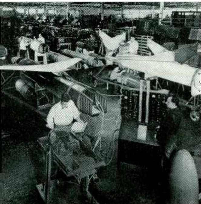
The Navy's new Martin KDM-1 pilotless target drones come off the sleepless Baltimore production lines. Powered by ram-jet engines, the target-drones are remote-controlled by radio and tracked by radar, to simulate the flight of an attacking airplane
