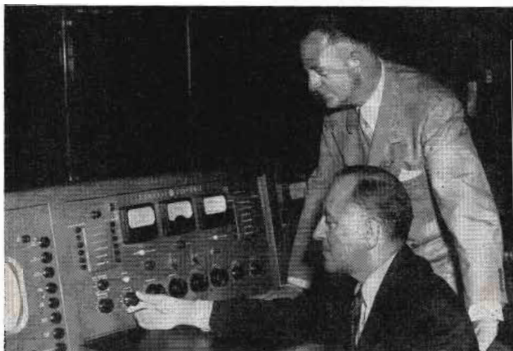
As forty TV stations increase their radiated power, J. R. Poppele, vice-president and chief engineer, WOR-TV, New York, and Charles H. Singer, assistant chief engineer, are shown turning up WOR-TV's ERP from 9 kw to 22 kw
