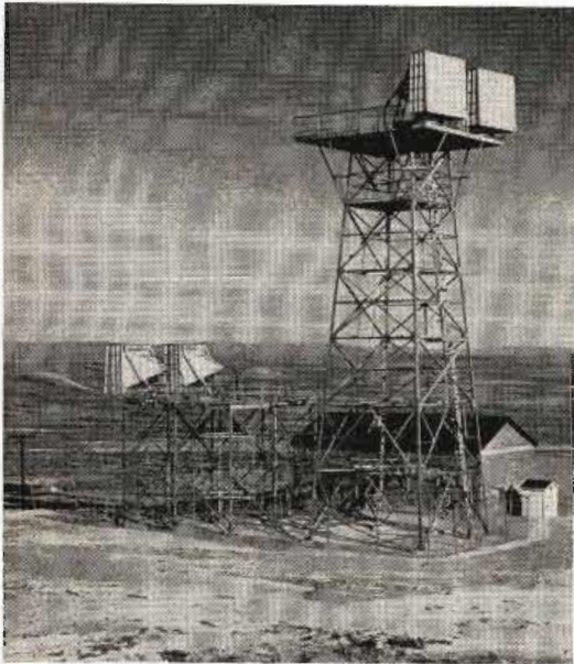
Microwave relay transmitting and receiving antennas are at different heights in Creston, Wyoming installation where the TD-2 system crosses the Continental Divide
