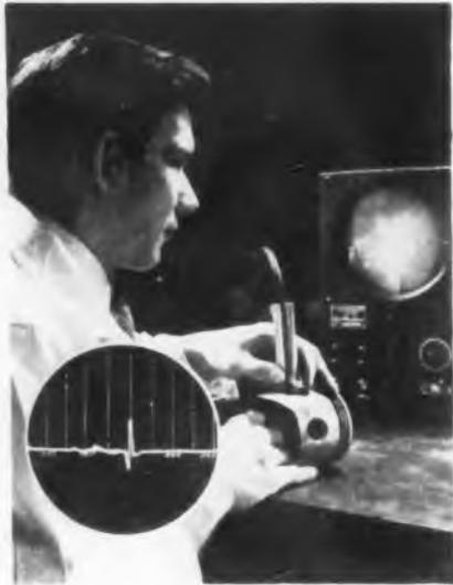
GM-developed Sonigage utilizes ultrasonic resonance to measure thickness and detect internal flaws. Inset shows vertical trace deflection on CRT for measuring 0.07 in. steel
