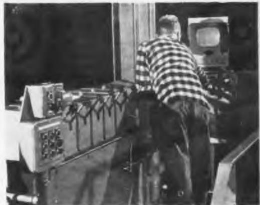
From 300 feet inside Ford stamping plant, operator uses TV screen to observe loading of steel trimming bales into waiting freight cars
