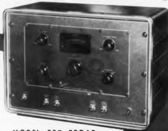
**MODEL 907 BROAD-BAND SWEEP FREQUENCY GENERATOR** - A fundamental oscillator which can be swept over a band not less than 8 Mc/s for center frequency of 40 Mc/s. Sweep width not less than 40 Mc/s over the UHF band. Output continually variable over voltage range of 10  $\mu$ v to  $\frac{1}{2}$  volt.
