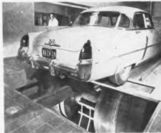
Rear wheels of auto turn drums coupled to dynamometer measuring speed-torque characteristics. Westinghouse electronic controls simulate wind resistance and road grades
