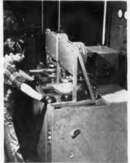
GE automatic induction heat and quench at Chrysler. Hardening depth is controlled to 0.015 in. Type 880 triode is used in oscillator
