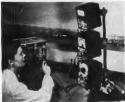
instruments easier to attach, adjust, and read. Multiple ac outlets are provided in the base for instrument power cords. The mounted instruments shown are the model 301 audio oscillator (range 10 cps to over 1 MC), model 401 high resistance bridge (100 k to 100 megohms, 0.25%), and the model 201 vacuum tube voltmeter for dc, ac, and resistance measurements. **Beckman Instruments Inc., Shasta Div., P.O. Box 296, Sta. A, Richmond, Calif.—TELE-TECH & ELECTRONIC INDUSTRIES.**
