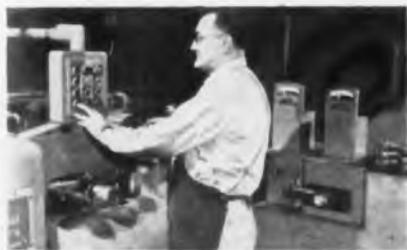
Electronic weighing machine automatically sets milling machine if Ford connecting rod and cap assembly are not in static balance. Cutters then remove metal to achieve balance within 2 grams
