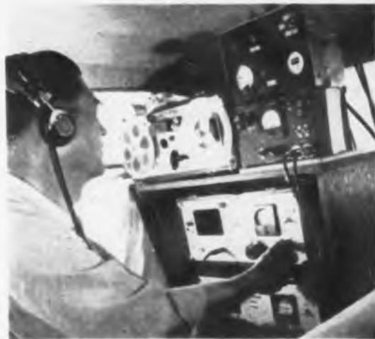
Magnecord tape recorder stores sounds picked up by microphones strategically located on moving car. Playback in laboratory will permit further analysis
