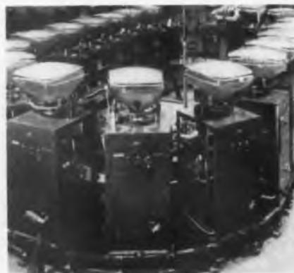
tions and can be converted to the inline system when additional capacity is needed. The stationary, or bench type unit is suited for color TV tube leak-checking without major alterations. Cycling is automatic. **Consolidated Vacuum Corp., 735 Ridge Road West, Rochester 3, N.Y.—TELE-TECH & ELECTRONIC INDUSTRIES.**
