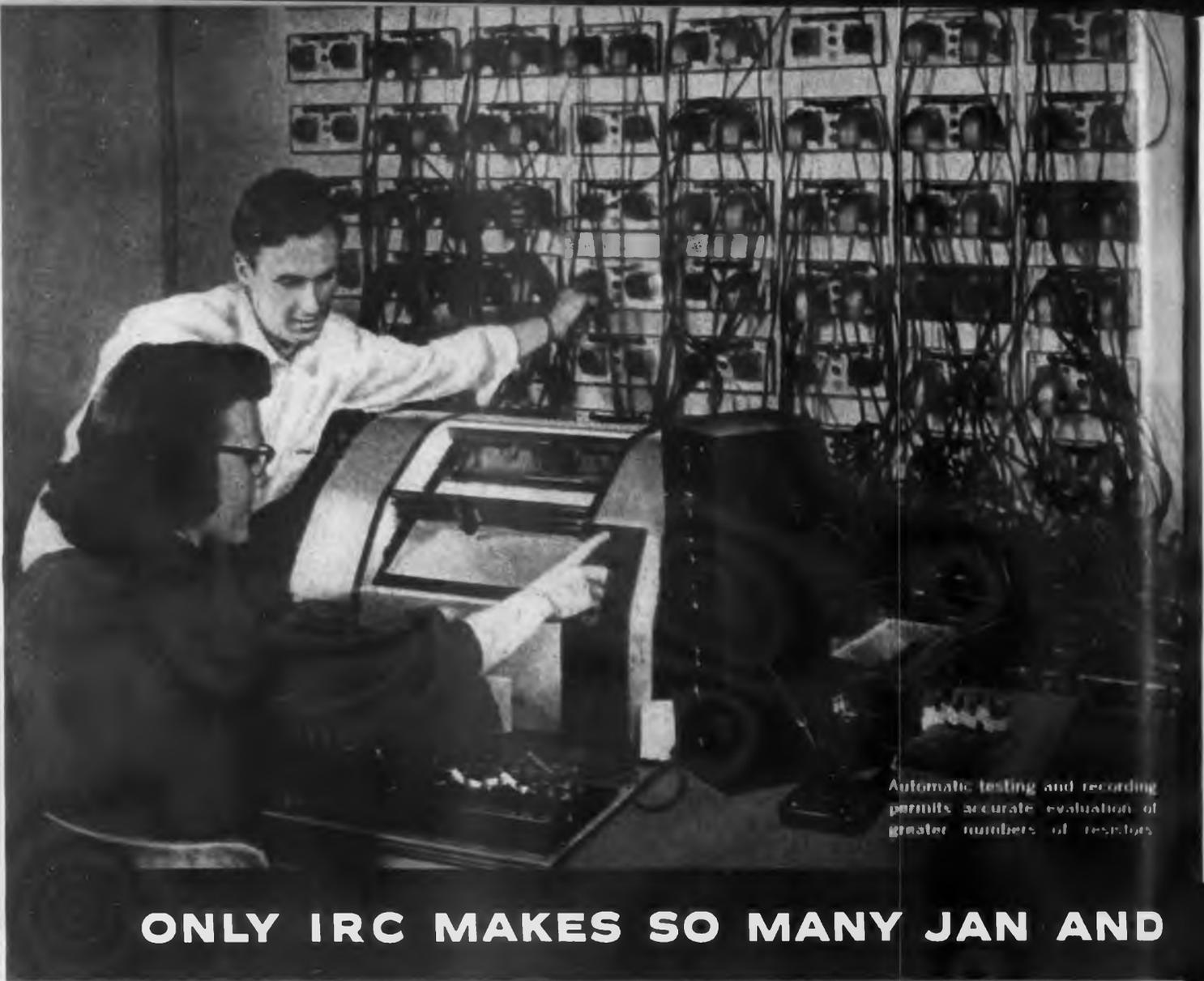
Automatic testing and recording permits accurate evaluation of greater numbers of resistors.
