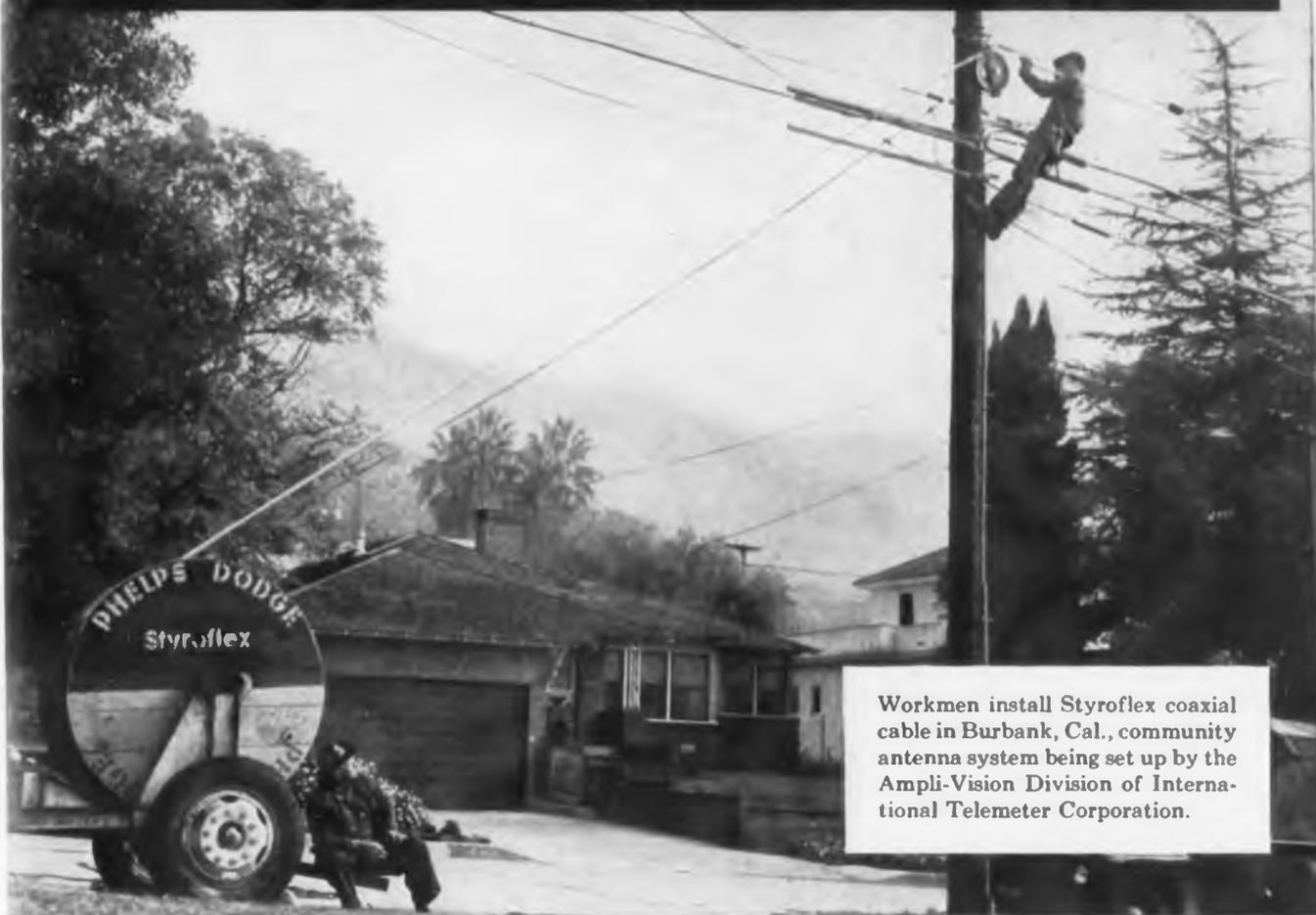
Workmen install Styroflex coaxial cable in Burbank, Cal., community antenna system being set up by the Ampli-Vision Division of International Telemeter Corporation.
