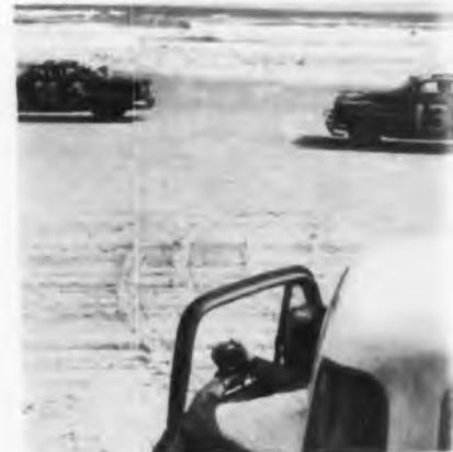
Two-way GE radio system serves as communication link between pit truck and two stock racing cars during 160-mile race at Daytona Beach, Fla. Lap, track conditions and gas supply information was relayed between drivers and pit
