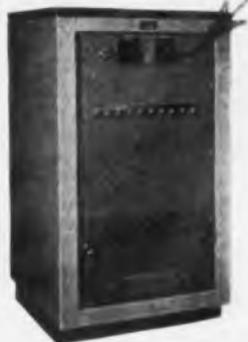
COMPLETE TRANSMITTER CONTROL IN UNDER-WINDOW CABINET
