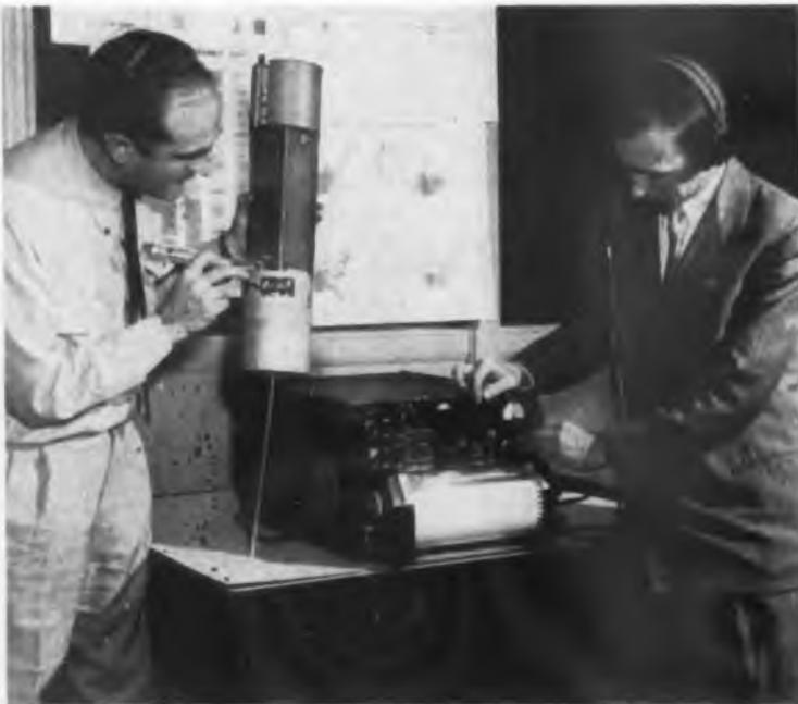
Wilson A. Maxim (l) and Donald A. Brown, engineers at Wright Air Development Center's Aircraft Laboratory adjust droppable radio-sonde (l) and airborne radio receptor (r), developed by WADC and Signal Corps. Equipment provides improved vertical atmospheric sounding information over ocean areas, wastelands and Arctic regions. Radiosonde transmits coded weather signals while falling
