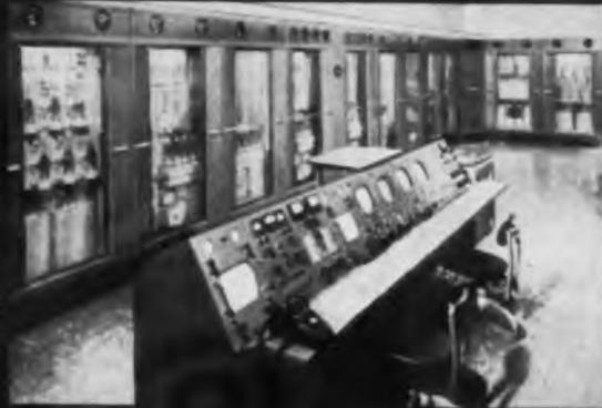
Transmitter room of WOR-TV's new Empire State 40 KW transmitter, 130 KW ERP, 100% air cooled. Completely self-contained. Equipment throughout by Standard Electronics.
