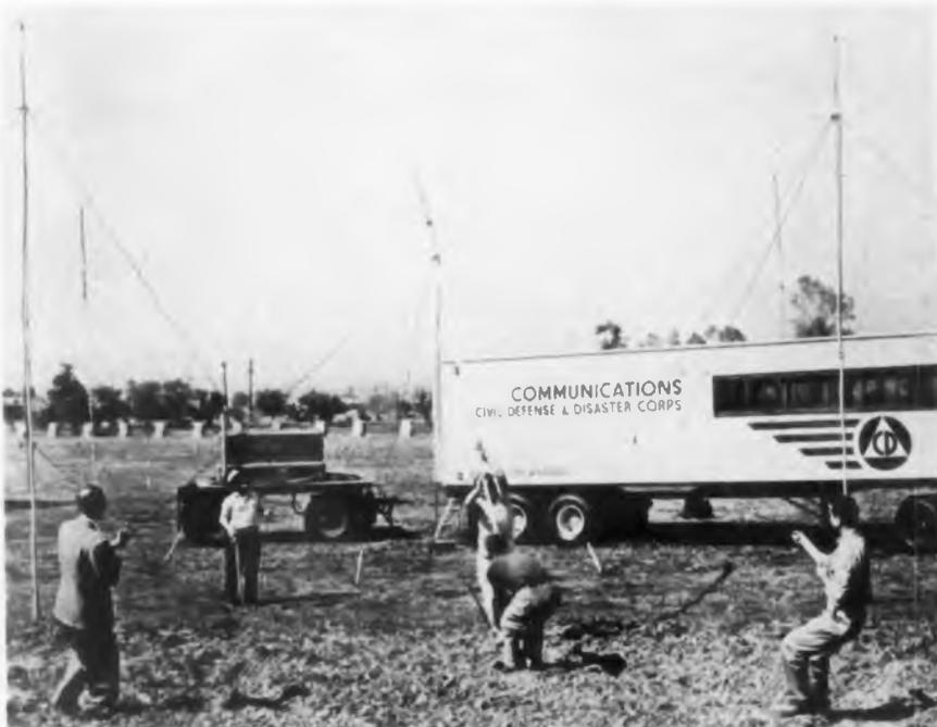
Los Angeles gears for Civil Defense communications with the addition of three new trailer-mounted mobile communications centers. The 35 ft. Fruehauf trailer houses six G.E. transmitters and receivers with working space for station operators. The units, which cost approximately \$40,000, are linked to 36 fixed communications centers throughout the city. The entire system requires 17,800 persons
