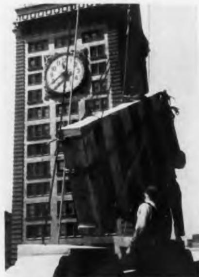
One of Remington-Rand's famed Univac's is delivered to Metropolitan Life Ins. Co. in N.Y. Parts of the electronic computer were so bulky that they had to be lifted by hoist to 20th floor
