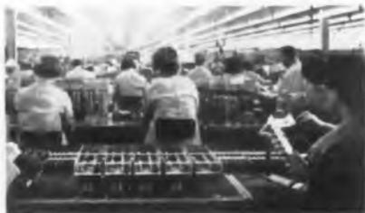
The new home of C. P. Clare & Co., relay manufacturers, at 3101 W. Pratt Blvd., Chicago, was designed to eliminate the dust and dirt that cause the majority of electrical relay failures. Temperature and humidity controlled air is circulated through the plant after passing through a bank of self-cleaning electronic precipitators
