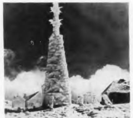
This is how the TV antenna atop Mt. Washington, N. H., looks in winter. New installation under construction for station WMTW-TV will employ Caterpillar diesel electric sets to provide power to de-ice tower in the -40° zone
