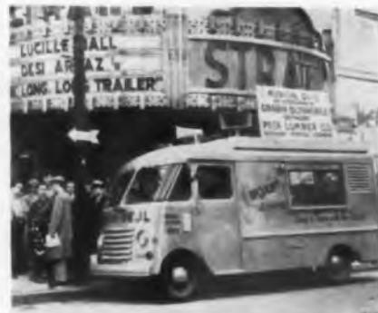
This unit used by WQAN, Scranton, Pa., is a self-contained broadcasting station with high frequency transmitters, tape recorders and audio equipment, as well as public address equipment all powered by a gasoline engine generator.
