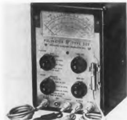
17 megohms, shielded ac and r-f leads, and screw-on connectors. Reads peak-to-peak voltages from 200 mv to 2,800 v; dc voltages from 200 mv to 2,800 v; dc voltages of plus or minus polarity from 50 mv to 1,000 v; ac voltages from 50 mv to 1,000 v, r-f voltages from 100 mv to 300 v in the band of 10 kc to 300 mc. Sylvania Electric Products Inc., 1221 West Third St., Williamsport, Pa.—TELE-TECH & ELECTRONIC INDUSTRIES.
