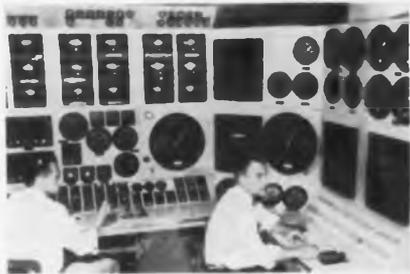
From this control room, protected by two-foot concrete walls, engineers run dynamic tests on jet engines. Engineers of Ford Aircraft and Minneapolis-Honeywell collaborated on the work
